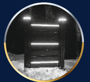
LED lighting - p. 47
